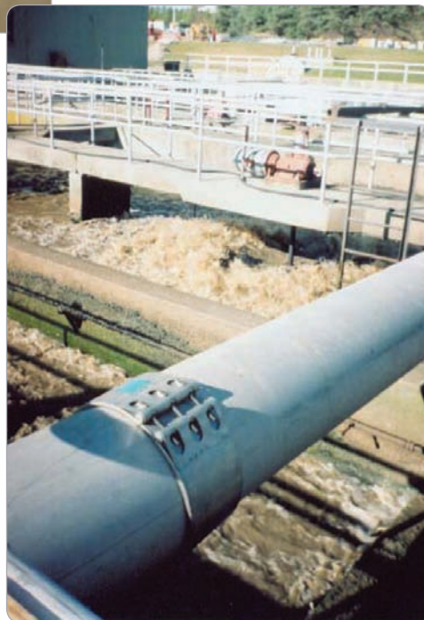
48" (1200) YN MF-RL Expansion Coupling on Air supply header from bolwer building. Some couplings were used in Lieu of field welding
