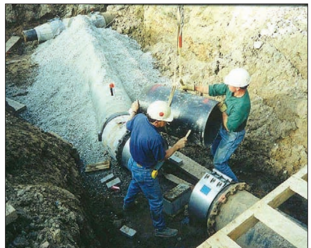
▲ UNDERGROUND REPAIR PIPELINES
